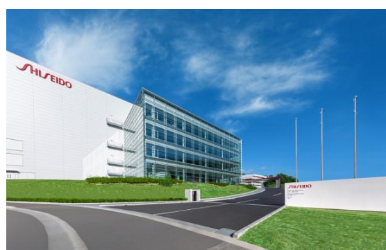
Osaka Ibaraki Factory and West Japan Distribution Center
